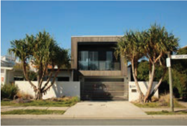
Flat Roofs (Vertical)
